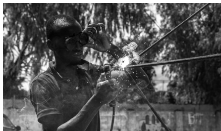
Fig. 5: A local welder man is giving the final touches to a Bantaba (garden pavilion) co-created by youth during the Weld Champions workshop in Soma.
