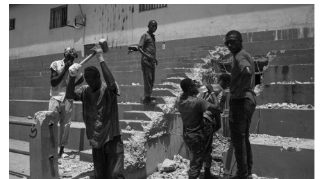
Fig. 6: The first intervention of Building Together was to create a connection between the study café and the basketball court at the youth centre in Basse.
