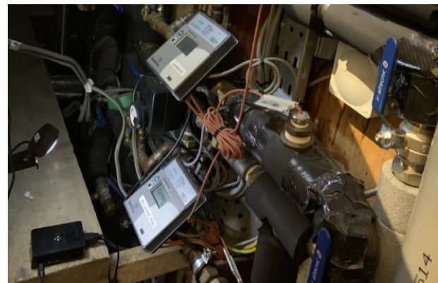
Fig. 11. Heat meter arrangement in the Helix building.
