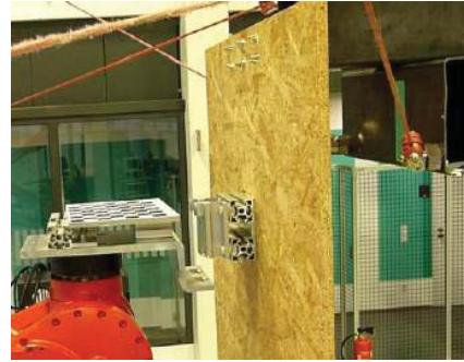
Fig. 4: Demonstration of a panel installation with a CDPR
