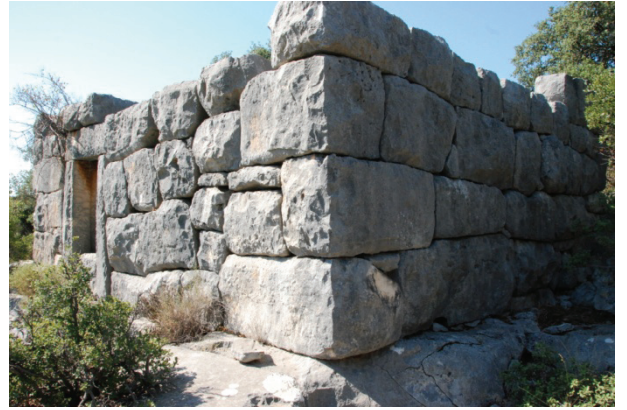
Fig. 2: The tower building of a square plan at Kutluçakale
