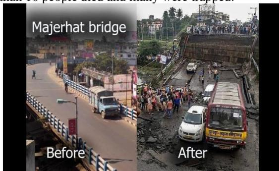
Fig. 1 The condition of the Majerhat bridge before and after the collapse in Kolkata
