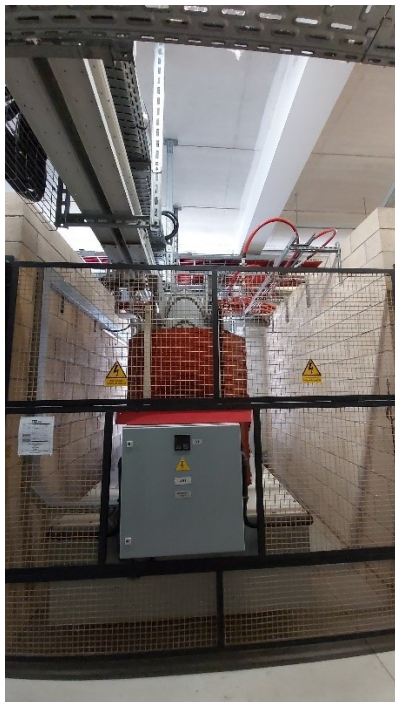
Figure 21: Transformer cabinet for MV measurements at CENER.
