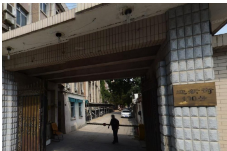
Main entrance of the Institute, 100 Yingxin Street—2020
