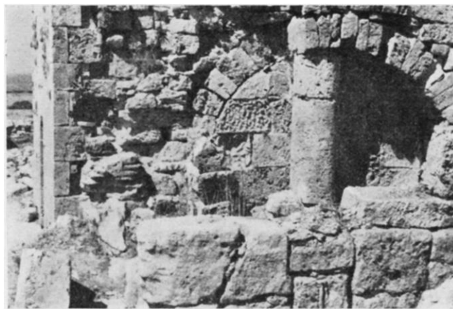
FIG. 9.—APHENDRIKA, PANAYIA. COLUMN OF SOUTH COLONNADE REMAINING in situ .
