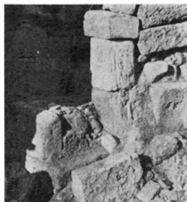
FIG. 14.—SYKHA, PANAYIA. EAST HALF-COLUMN OF NORTH COLONNADE.
