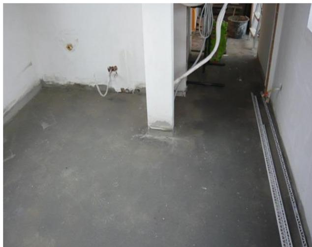
**Figure 4.** Installed floor screed with recycled AAC in a case study in the Port of Antwerp.
