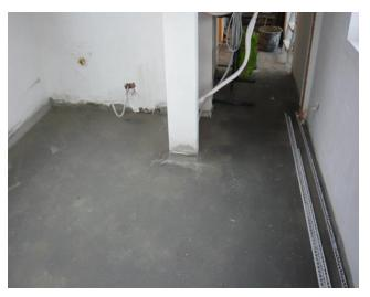
Figure 4. Installed floor screed with recycled AAC in a case study in the Port of Antwerp.
