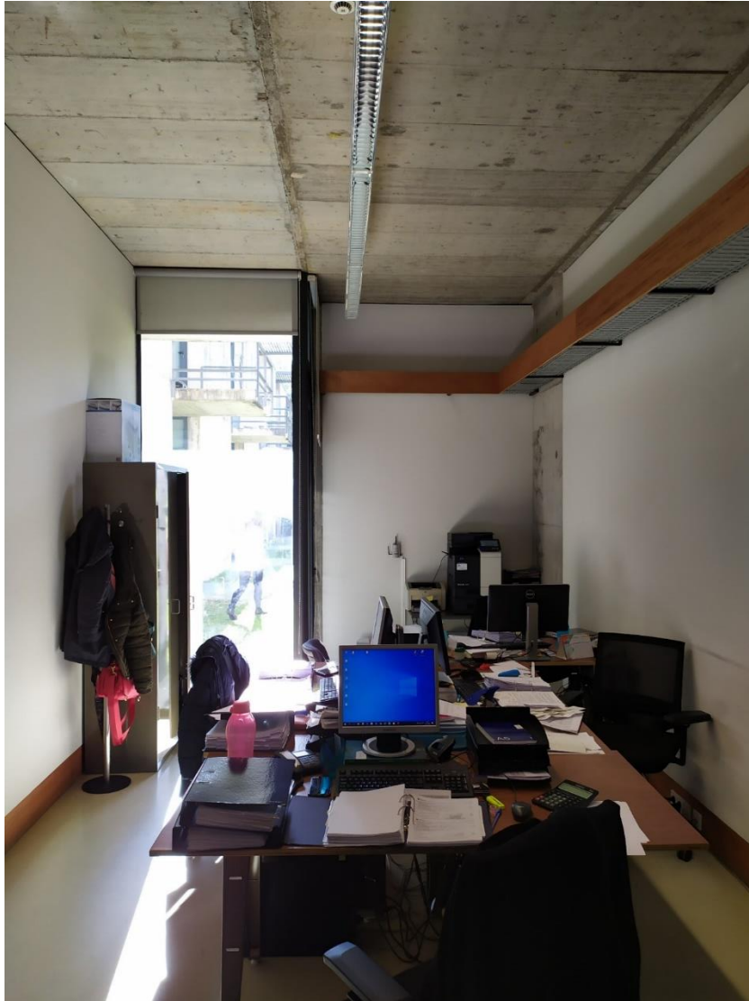
FIGURE 14: IPN BUILDING C (SOUTH FACADE) – OFFICE
