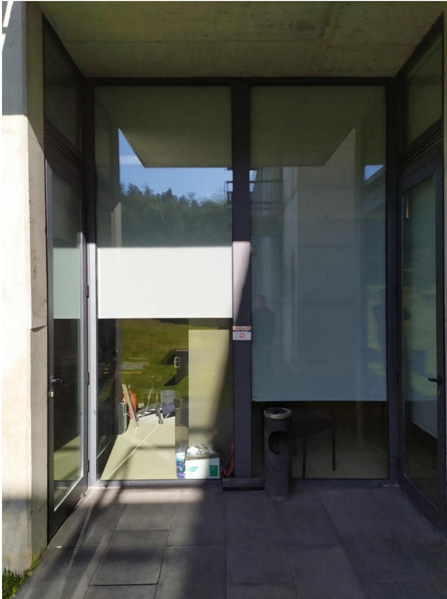
FIGURE 13: IPN BUILDING C (SOUTH FAÇADE) – OUTSIDE WINDOWS AND DOORS
