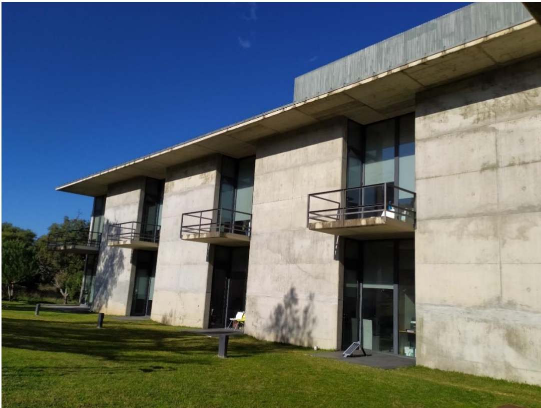
FIGURE 12: IPN BUILDING C (SOUTH FAÇADE) – PROPOSED LOCATION FOR THE DEMO
