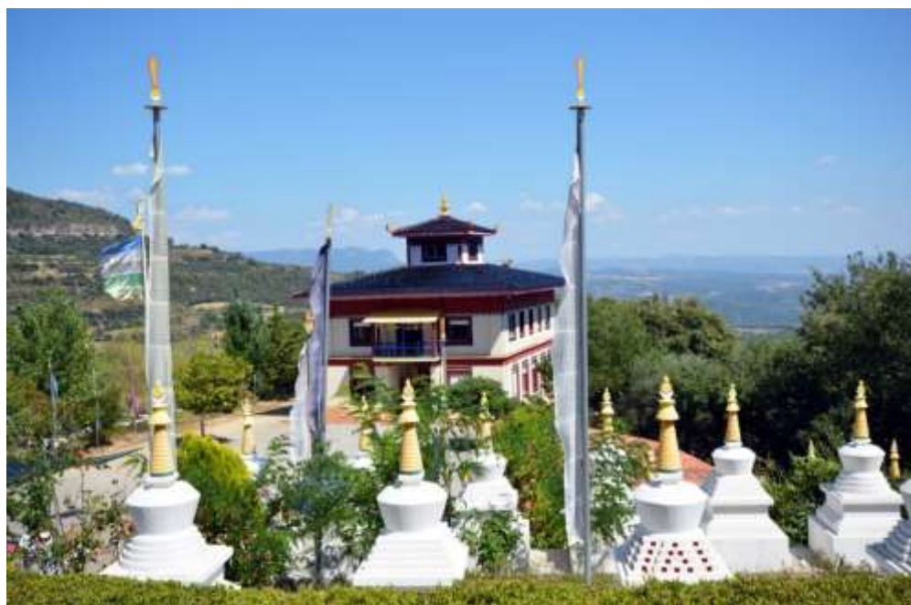
Illustration 43: Dag Shang Kayu. Building of the meditation hall (view from the main stupa)
