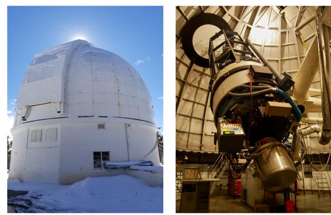
Left: Dome enclosure for Boston University's Perkins Telescope Observatory (PTO) at Anderson Mesa Station, near Flagstaff, Arizona. Right: Interior of the PTO, showing the 1.83-meter Perkins Telescope with the Mimir instrument (Clemens et al. 2007) mounted on the back. PINES uses Mimir in its wide-field (10'x10') *J*- and *H*-band imaging modes.
