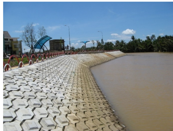
Fig. 1. Shell concrete block mat for seacoast protection.
