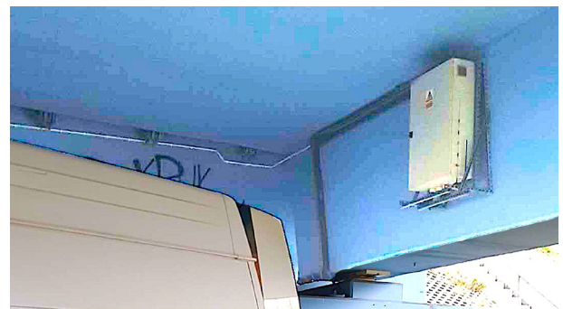
Fig. 8 Protection box under bridge
