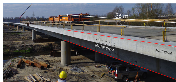
Fig. 3 Monitored bridge span of Gm1-2W at Southeast end
