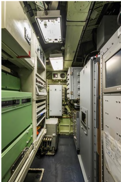
Figure 5: Electronic Hut After Conversion
