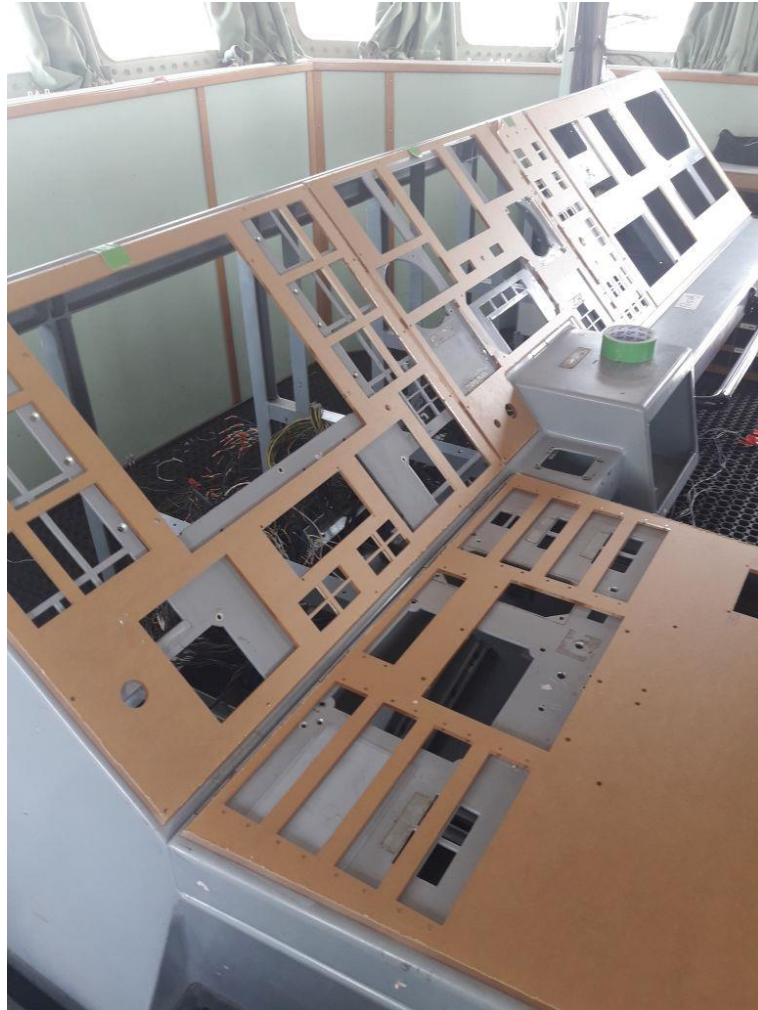
Figure 5. Templates being assessed on the existing Bridge Console Chassis
