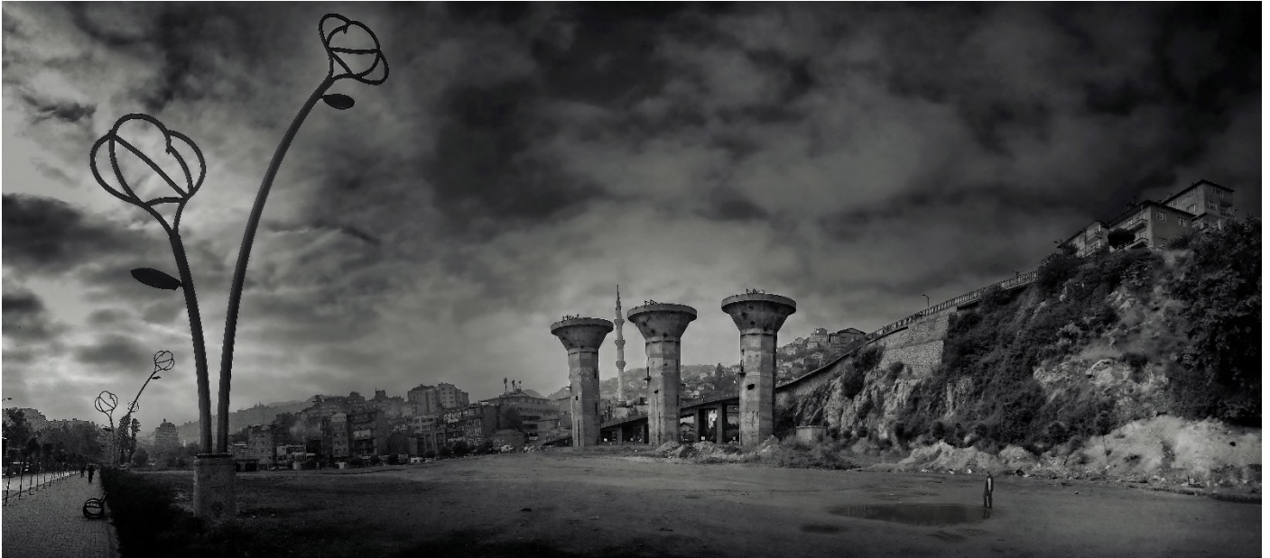
Zonguldak: Lavuar coal-washing plant after demolition, early 2010s.
