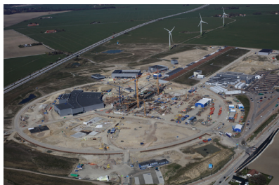
Figure 1. ESS construction site, 2019 April
