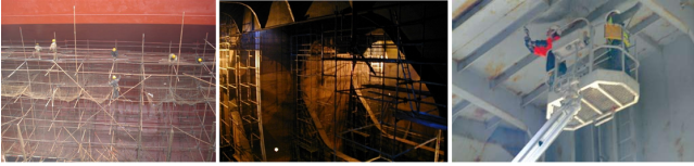
Figure 1: Access arrangements required during vessel inspection: scaffolding and cherry pickers.
