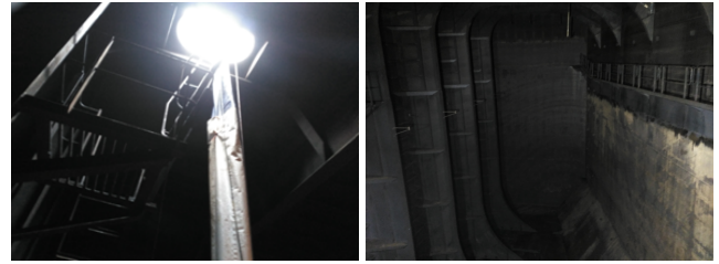
Figure 3: (left) Oil tanker manhole entry point. (right) Typical oil tanker cargo hold.
