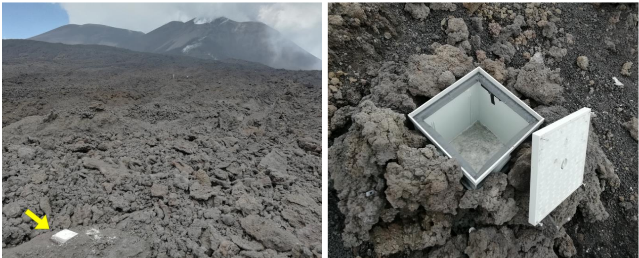
Figure 8 – Left: concrete base on Etna at 2900m elevation. The summit active craters are visible in the background. Right: bottomless PVC box, installed on Etna at 2600m elevation, in the framework of field-tests during the summer of 2019 (see Deliverable 3.2 for details). In the final setup, a PVC box different from the one shown here is utilized.
