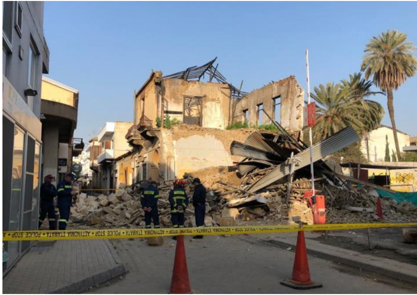
Derelict buildings in old Nicosia collapsing after heavy rains, 2019.
