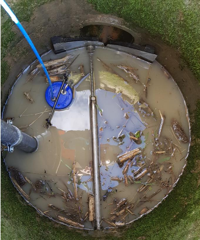
Figure S 3: Installation of a water-level proportional sampler in a storm drainage inlet.
