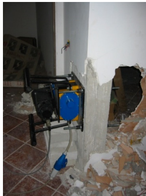
Figure 6. A vibrodyne on a Shear Wall.
