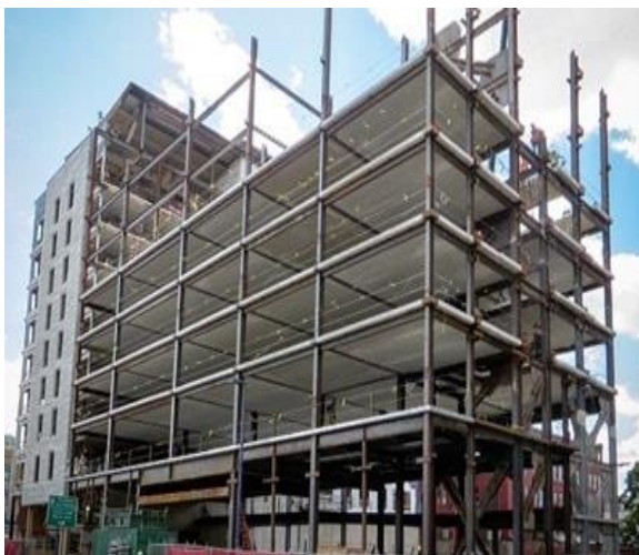
Fig.1:-Steel framed structure
