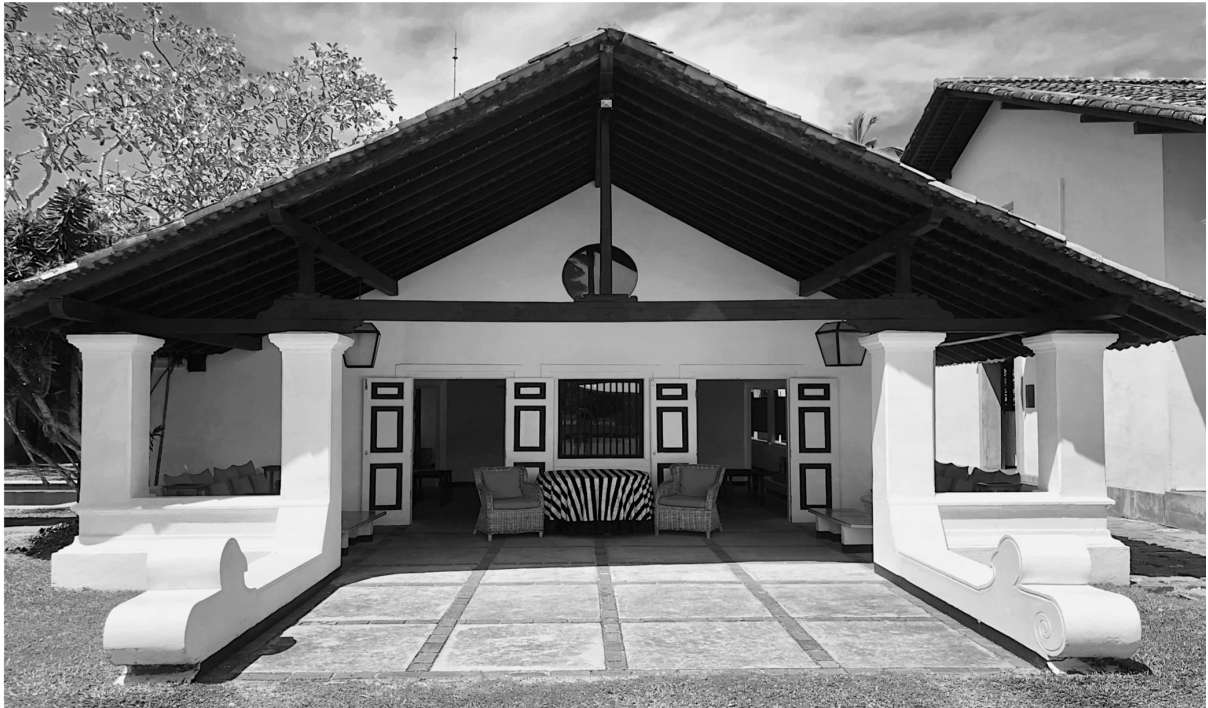
Figure 13: The west front of the initial villa- evident of the use of overhanging eaves and veranda permitting open flow. Photo by Jordan Wright.
