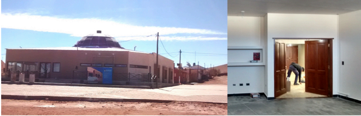
Figure 10: Operations and EPO building. On the left, perspective of the building. Right: view of the control room and laboratory.
