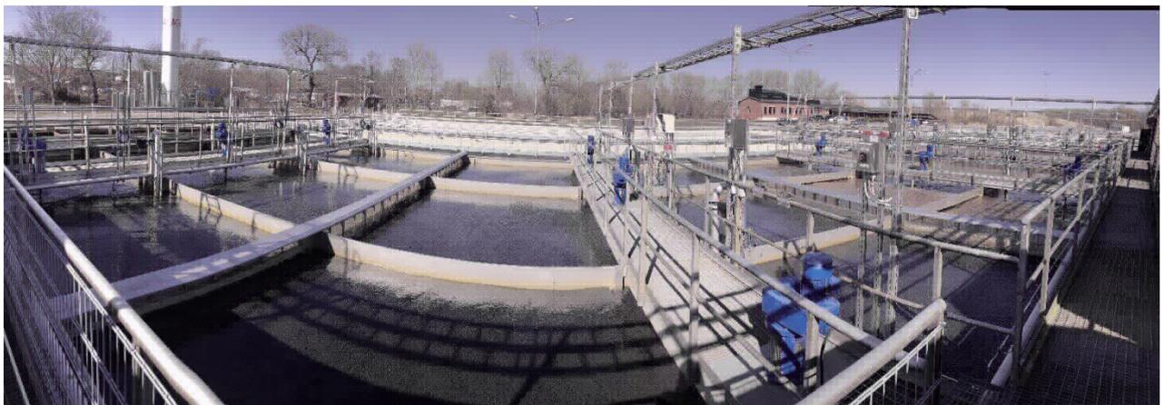
Figure 4: Panorama view of the MBBR plant in Linköping consisting of three separate lines with four reactors (2 x nitrification, 2 x denitrification) in each line.
