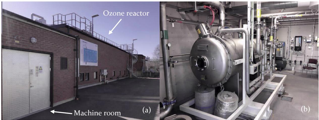
Figure 3: (a) Ozonation plant in Linköping. (b) Ozone generator model CFV30 from Ozonia.
