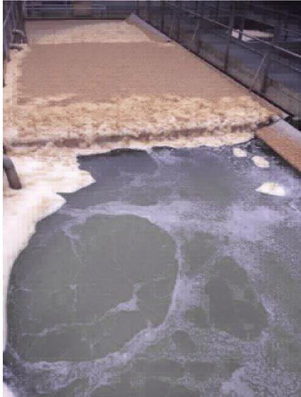
*Figure 26: Foaming in the ozone reactor effluent. Picture taken at the MBBR inlet compartment.*
