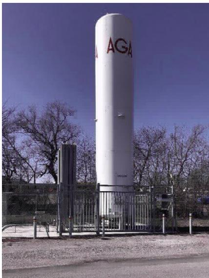
*Figure 27: LOX tank mounted on a concrete plate surrounded by gravel and grass for a safe work environment.*
