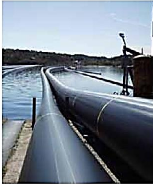
Continuous extrusion into the fjord
