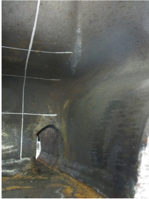
(e) South side K-area (West view)
