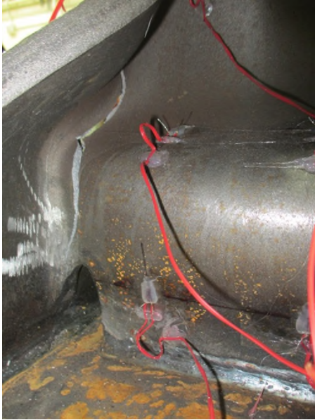
(e) South side K-area (West view)
