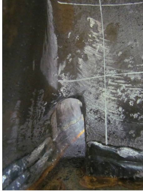
(e) North side weld access hole (West view)
