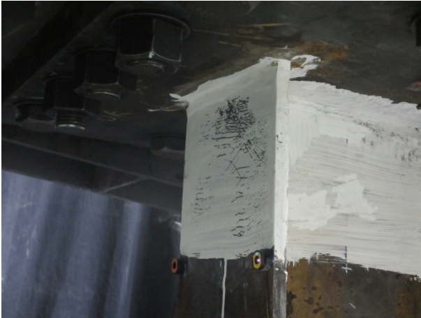
(e) Top end of north west flange
