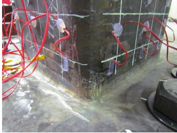
(a) HSS-to-base plate welding (H-27-C1-V)
