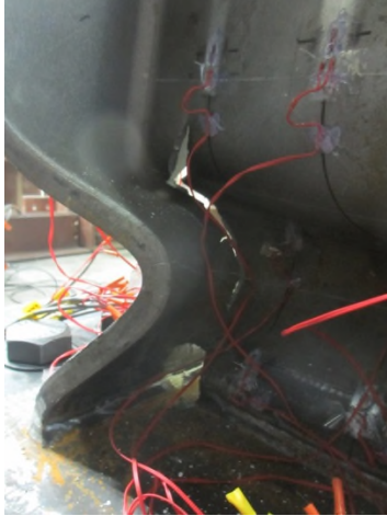
(e) South side K-area (East view)
