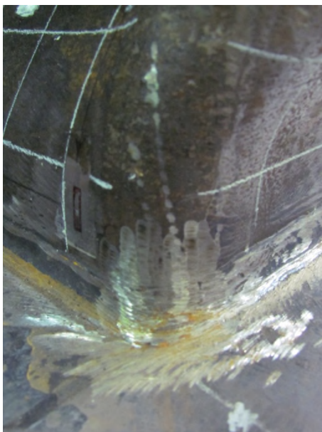
(c) Welding on north west corner
