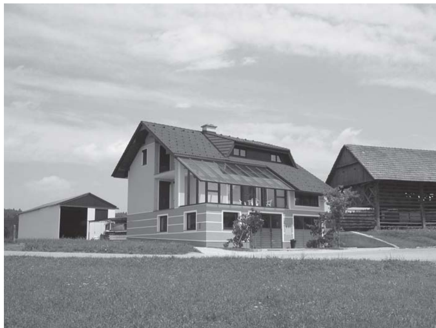
Figure 3.4 Typical example of a new single-family detached house in Ljubljana's urban region.
