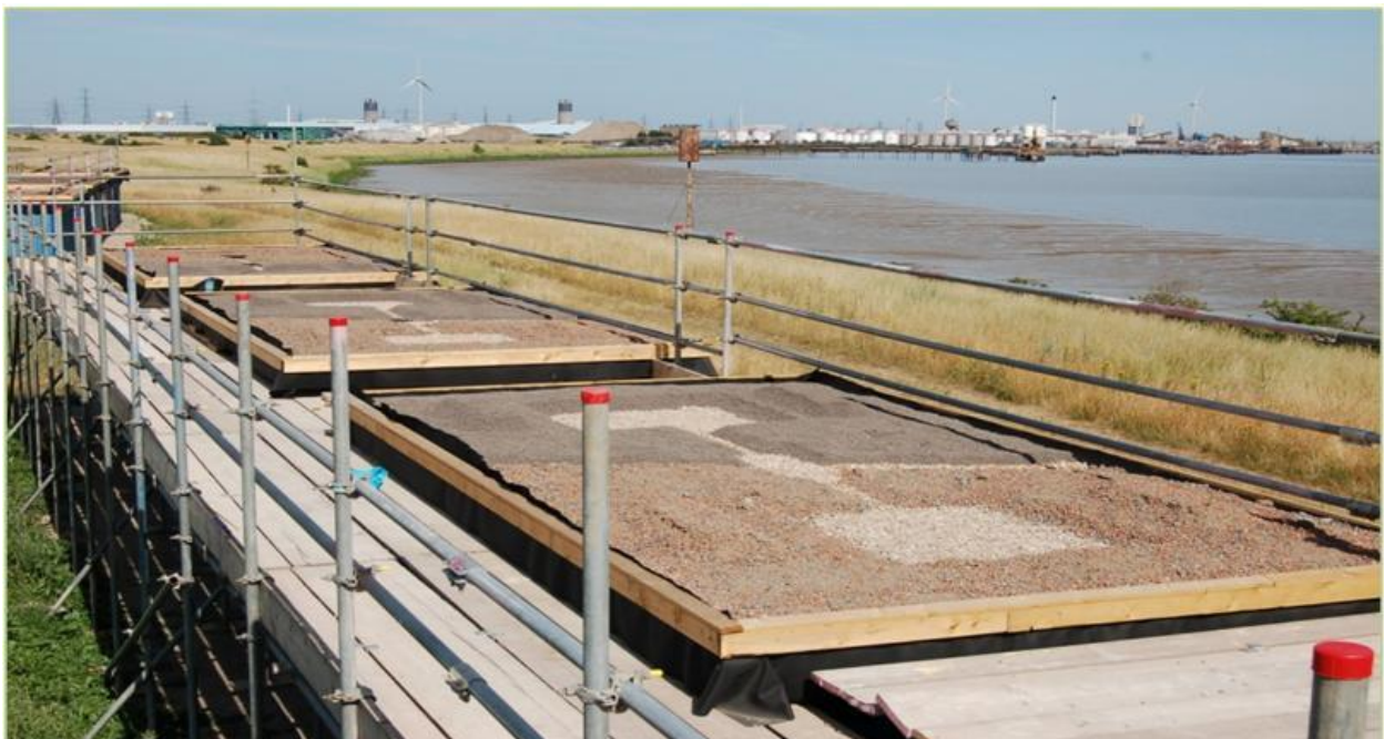
Figure 14. Construction of the Phase 2 green roof experiment at Barking Riverside offices
