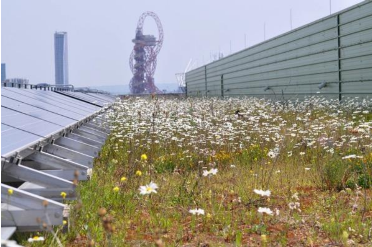
Figure 36. Biosolar (biodiverse green roof combined with photovoltaic panels) roof on the MPC building, Queen Elizabeth Olympic Park, London UK
