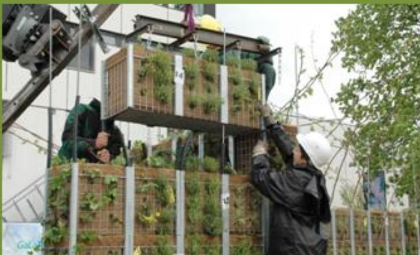
Construction of innovative multifunctional modular UGI
