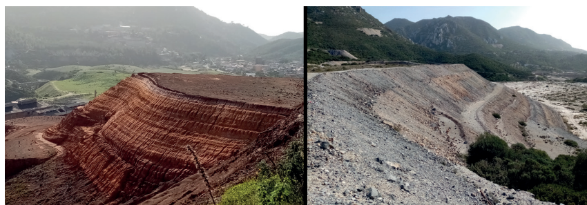
Figure 6: Extractive Waste Facilities. On the left Monteponi Mine red muds, on the right Masua Mine tailings pond.
