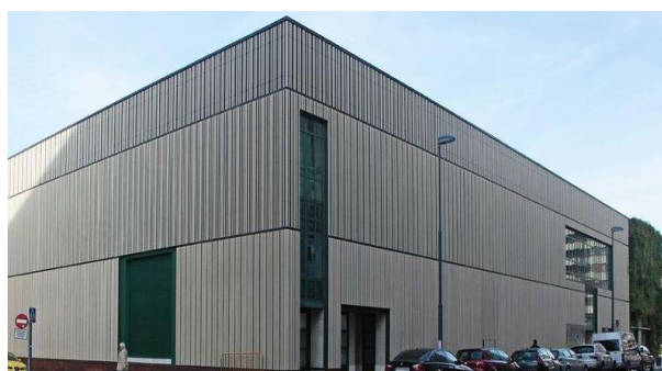
Figure 1: Façade of thermally modified Radiata pine, Madrid (a); Façade of thermally modified Eucalyptus, Segovia (b); Accoya interior panels, Google office Madrid (c); Accoya façade, congress palace Vitoria (d).
