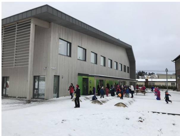
Figure 2: Chemically modified radiata wood cladding (Accoya) (a) and (b). Photo: Ostfold Research/Lars Tellnes.
