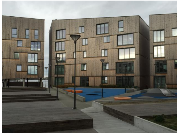
Figure 2: Vannkanten, Stavanger, Norge. Built 2014. Thermally treated pine (Delivered by Moelven). Photo: NIBIO/Lone Ross Gobakken
