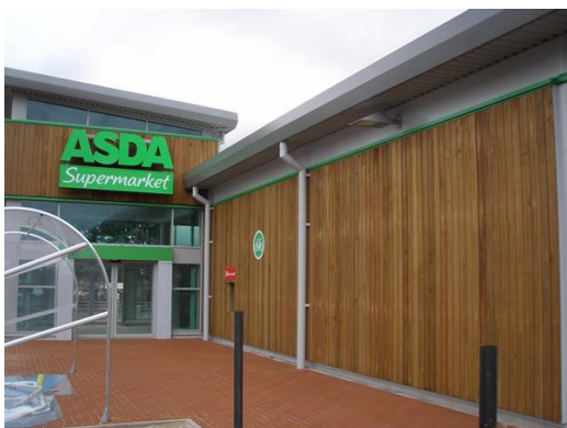
(a) Example of ThermoWood cladding, Telford
