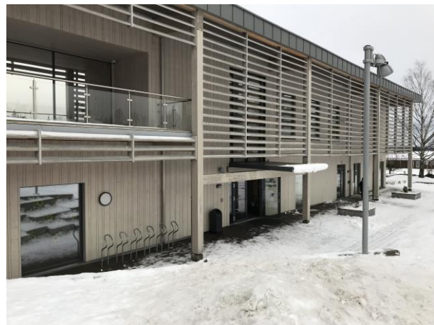
Figure 2: Chemically modified radiata wood cladding (Accoya) (a) and (b). Photo: Ostfold Research/Lars Tellnes.
