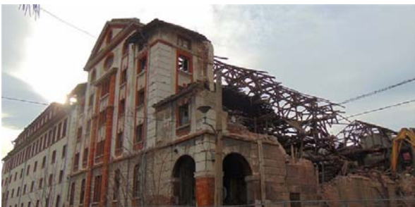
Fig. 7 The partially demolished tobacco warehouse [14]
