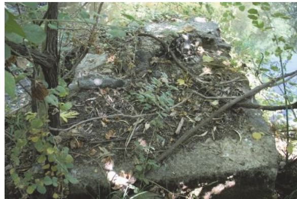
Fig. 28) Allıkavak Mevki . Remnant of a bridge pier
