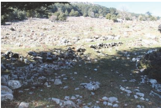
Fig. 13) Pinara – Telmessos. Retaining walls of the road in Akbel
