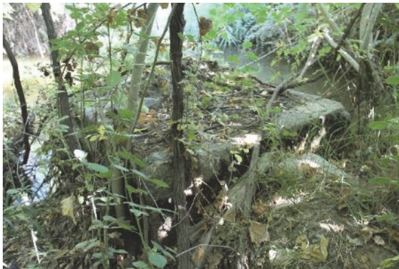
Fig. 27) Allıkavak . Remnant of a bridge pier
