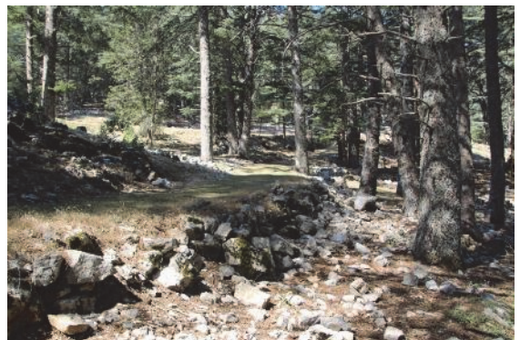
Fig. 14) Pinara – Telmessos. Retaining walls of the road in Akbel
