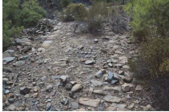
Fig. 32) Paşadöğüşlü. Road pavement
