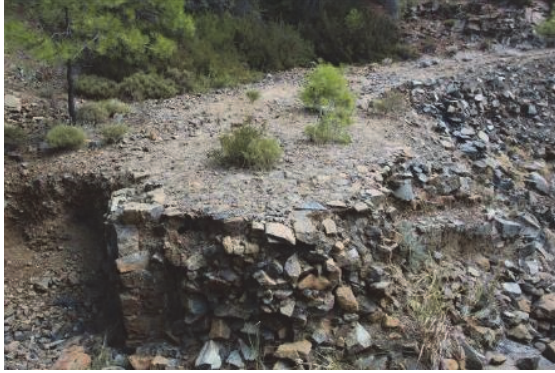
Fig. 31) Paşadöğüşlü. Road pavement
