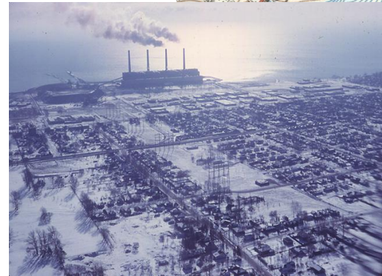
Image courtesy: "4 Sisters' and their Demolition!" Insauga . March 27, 2016. https://www.insauga.com/the-4-sisters-and-their-demolition
