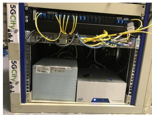
Figure 8: 5GCity Edge/MEC nodes at BeTeVe. L2/L3 Router Cisco ASR920 (top), Edge Server 1 and Edge Server 2 (at the bottom of the minirack).
