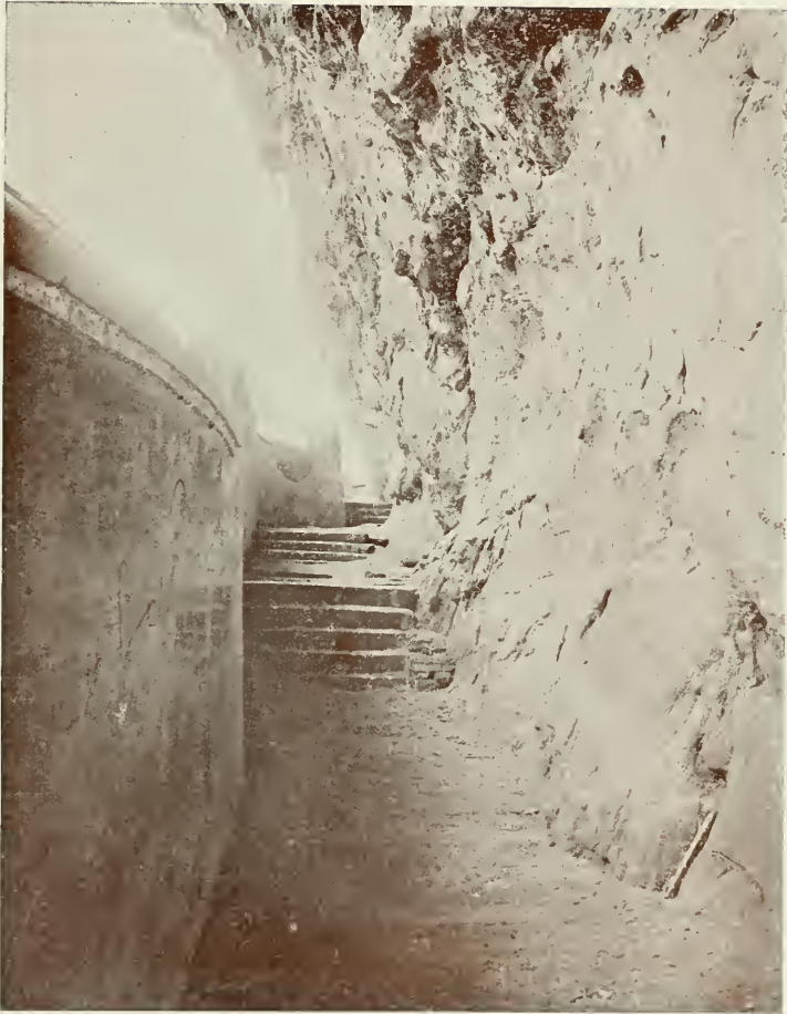
Archæological Survey photo.
