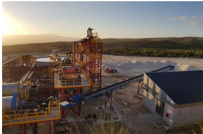
Figure 15 Image of the gravimetric plant
