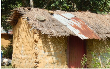
Fig. 28. — Traditional termite house. © E. Miabangana.
