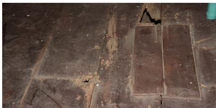
Figure 6. Wooden flooring. Source: Tolentino, R.P.G.
