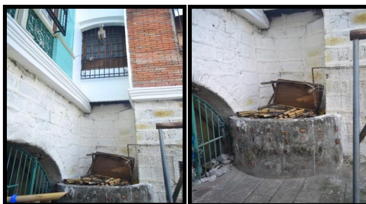
Figure 9. The rear of the structure with Balon . Source: Tolentino, R.P.G.
