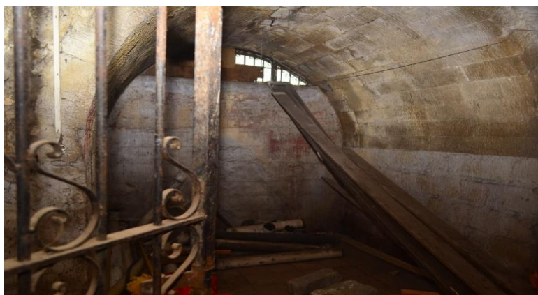
Figure 10. Arch room turned into bodega
