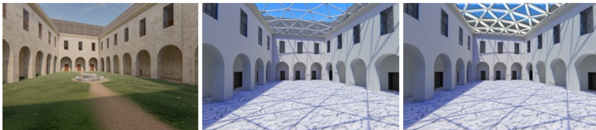
Figure 1. Left picture (Variant A): original atrium before renovation; middle picture (Variant B): renovated atrium covered by ETFE foils; right picture (Variant C): atrium after renovation covered by glass.
