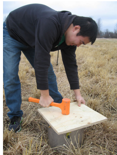
Figure 15. Installing the chamber
