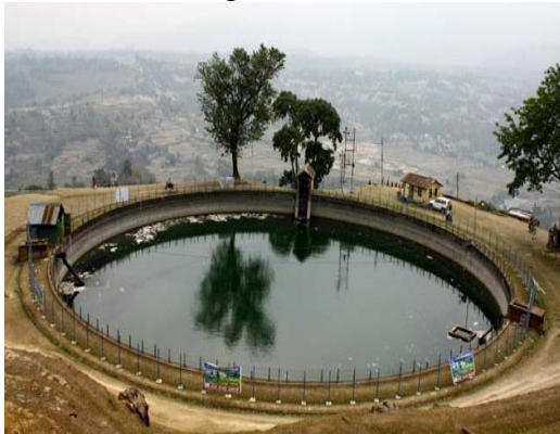
Fig.2:-Reservoir of the Pharping Hydropower Station
