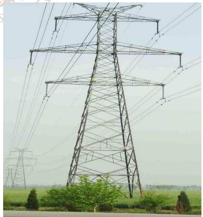
Fig1.1. Transmission line tower
