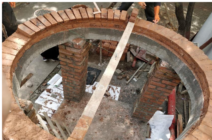
Figure 4: Tool (wooden flat log) used for maintaining the levels and center of each layer.
