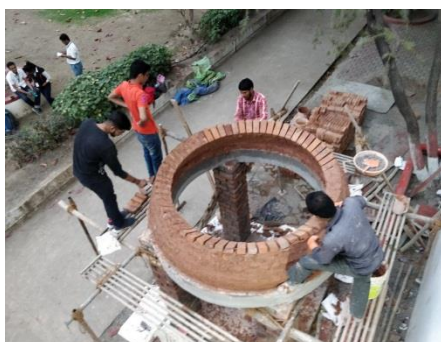
Figure 6: End of construction at day 2.
