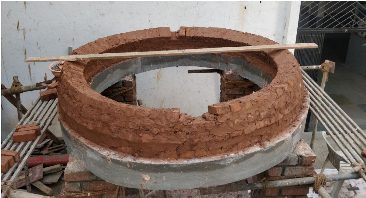
Figure 5: Masonry dome under construction without using formwork.
