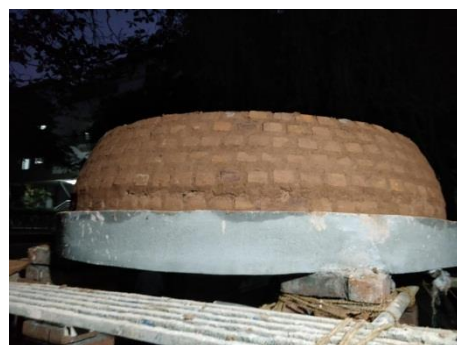
Figure 7: Top view of the dome under construction.
