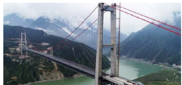
Fig. 7 Xingkang Bridge (open source image)
