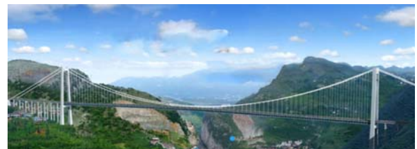
Fig. 6 Chishuihe Bridge (open source image)
