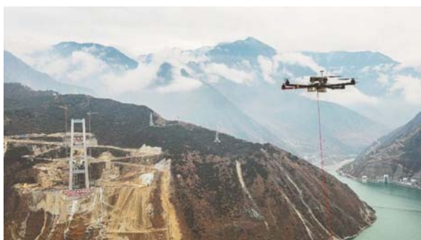
Fig. 9 Drone carrying the first pilot line between the towers [55]
