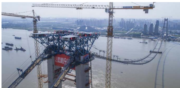
Fig. 8 Yangsigang Bridge (open source image)
