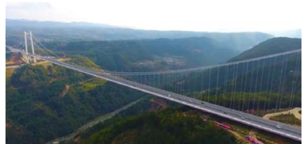
Fig. 5 Longjiang Bridge (open source image)
