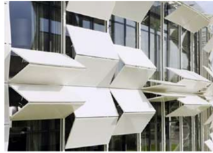
Kiefer Technic Showroom, Austria
