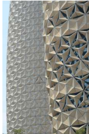
Al-Bahar Tower, Abu Dhabi
